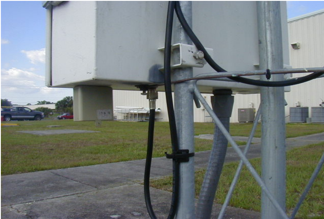
Illustration – Ground wire connected to RTU Polyphaser
